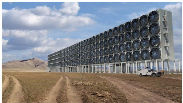
This artist's rendering shows Carbon Engineering's design for an 'air contactor' to pull carbon dioxide from the atmosphere.credit: Carbon Engineering
